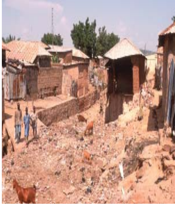
Figure 6: Buildings on drainage channels
